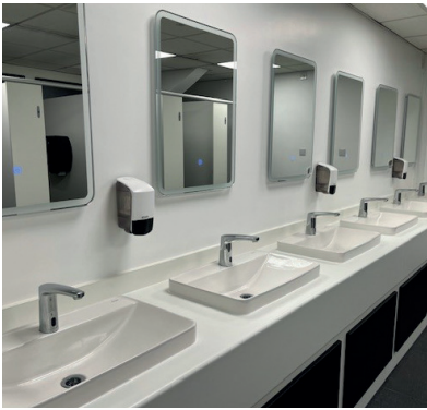
An infrared tap only runs when hands are detected, avoiding common issues of taps being left running, dribbling or overused. Inta produced and distributed 20,000 free copies of its Thermostatic Protection Guide , which explains how the risks associated with hot water systems can be managed
